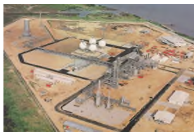
Onshore Escravos gas plant, helps to utilize Nigeria's gas potential and eliminate gas flaring. Photo by Chevron
