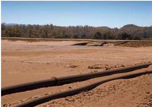
The cassiterite flotation tailing cover across the tailings at the start of the TSF rehabilitation in 1992.
