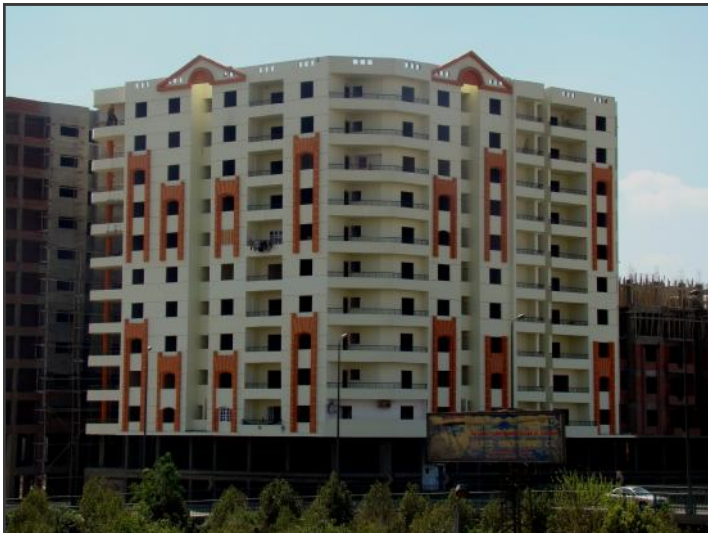
Figure 9: New Apartment Building under construction for 20 CORC Employees, May 2008.
