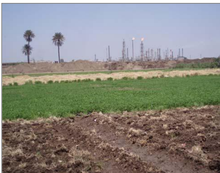
Figure 2: CORC Refinery, May 2008
