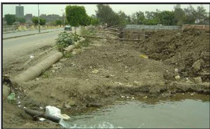
Figure 12: Groundwater Sampling Location
