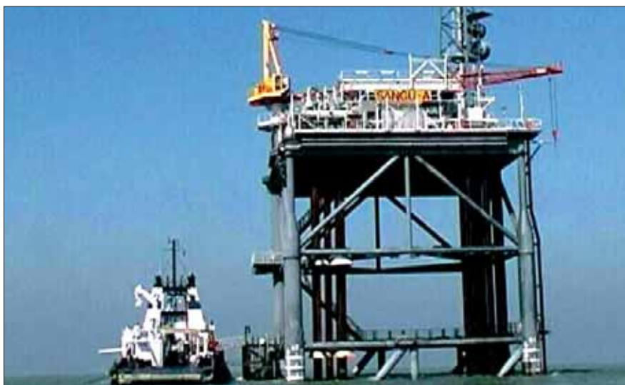
Sangu offshore gas platform
