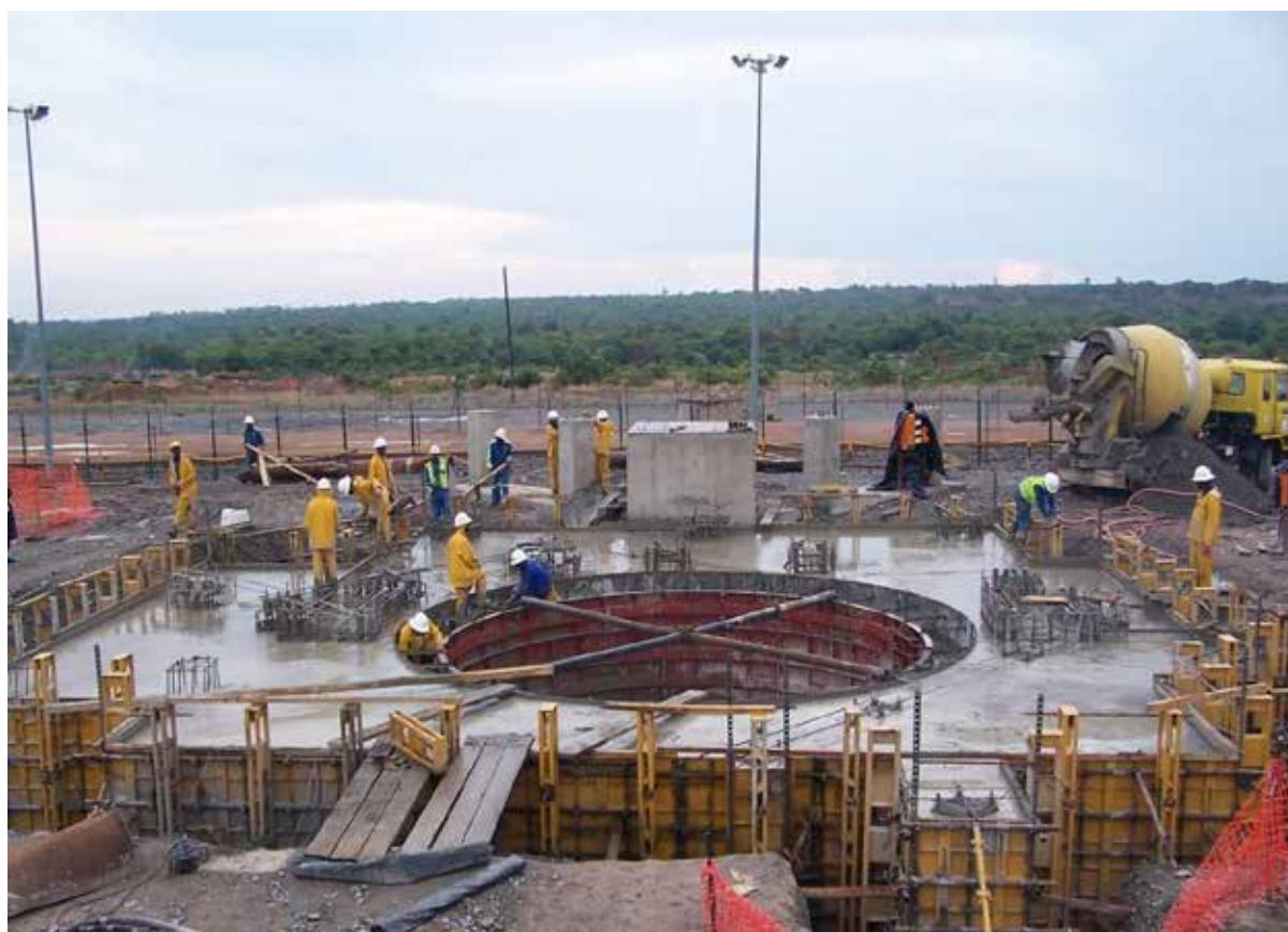
Construction of Synclinorium Shaft Collar
