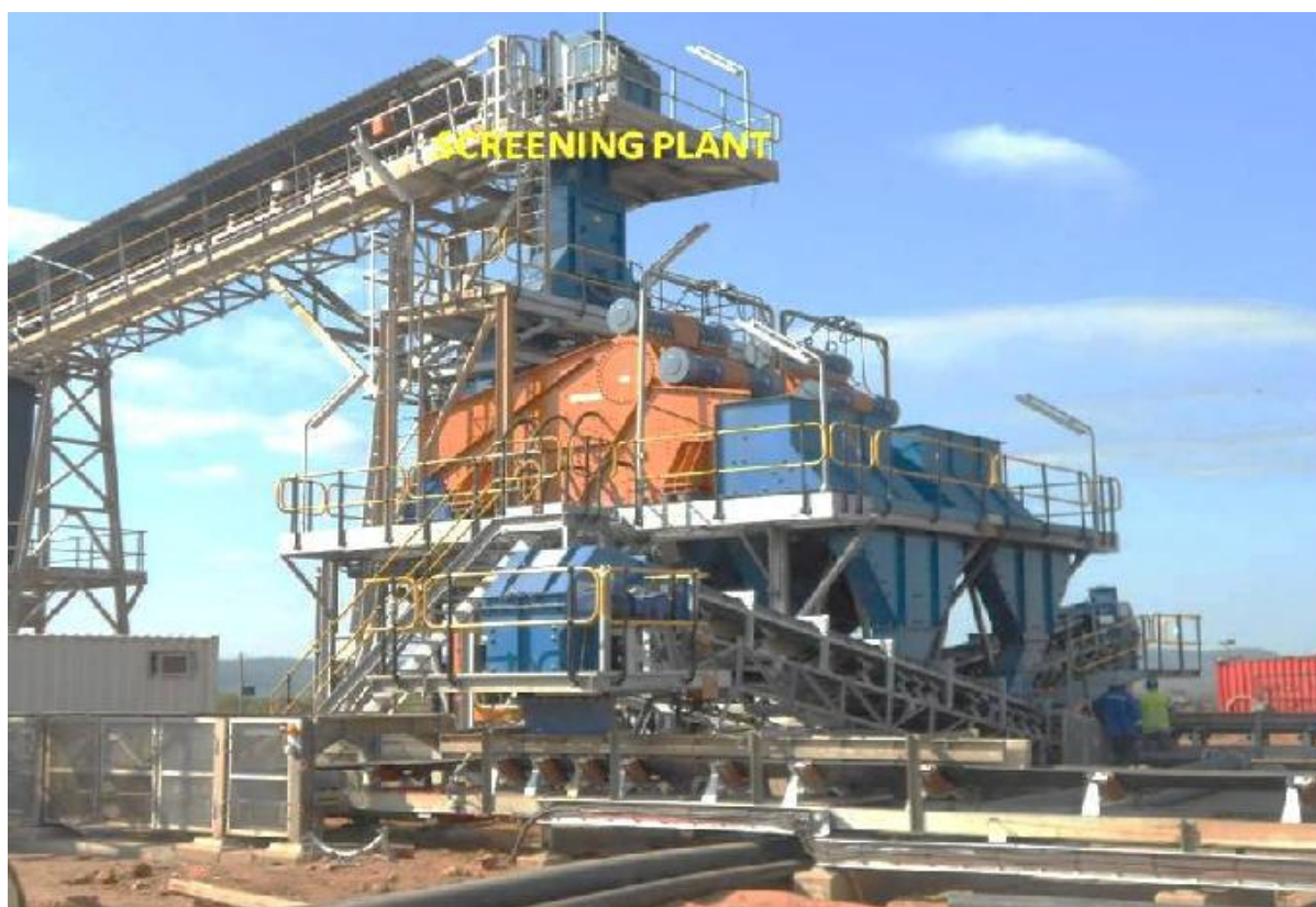
Parts of New Coal Handling & Processing Plant (CHPP)
