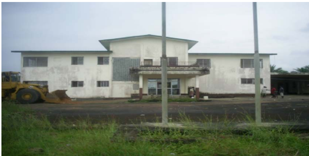
Presidential Palace Renovation for which US$59,796.88 was paid
