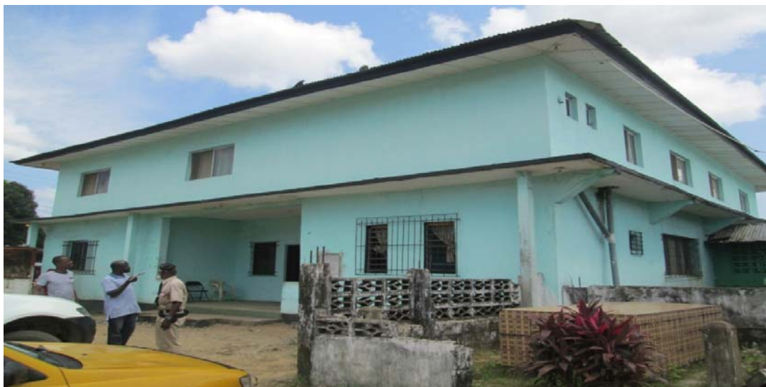
New Kru Town Library Project
