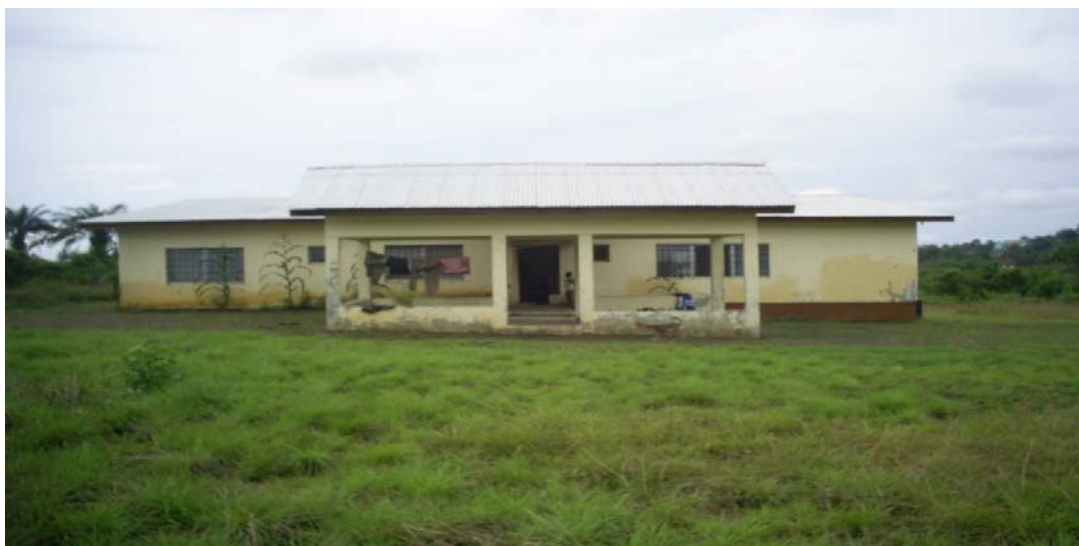
Careysburg Superintendent Residence Compound for which US$55,845.26 was paid
