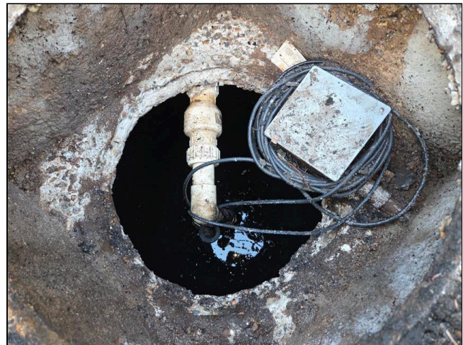
Pump chamber satisfactory
