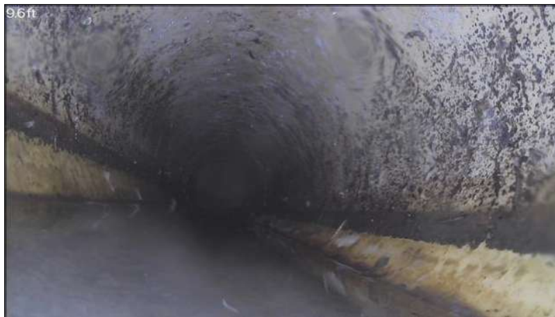
Sewer line intact
