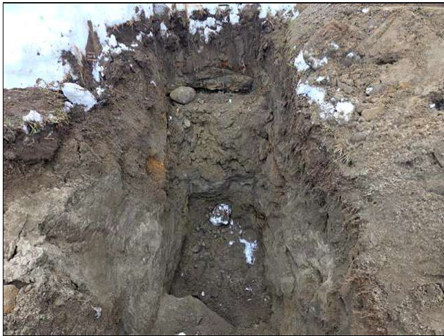
View of inspection hole
