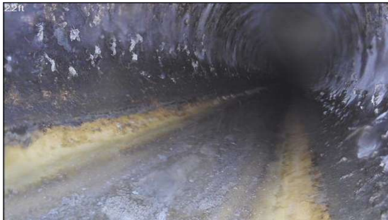
View of main sewer line
