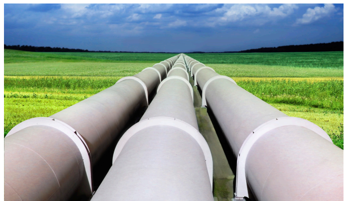
Pipeline applications make up a significant part of our experience in oil & gas.
