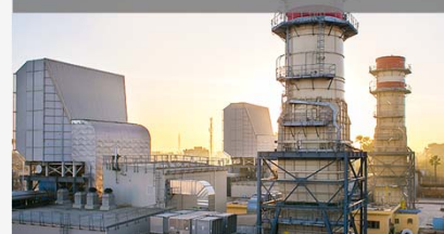
Mahmoudia Simple Cycle Power Plant Behira
