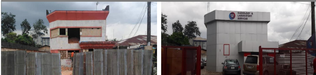
Benin Branch Renovation & Rebranding
