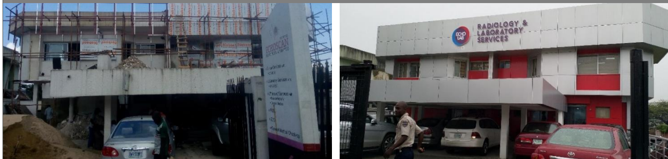
Opebi Branch Renovation and Rebranding
