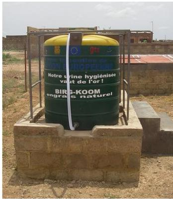
**Figure 5. Plastic urine storage tank in Ouagadougou, Burkina Faso installed as part of EU-funded project ECOSAN\_UE, Sept. 2008 (Photo: S. Rüd).**
