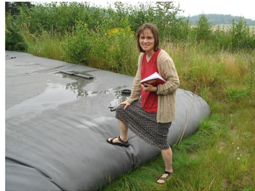
**Figure 6. Urine storage tank made of a PVC bladder (3 x 150 m<sup>3</sup>) at Lake Bornsjön near Stockholm (Sweden), Aug. 2007. Photo: E. v. Münch**
