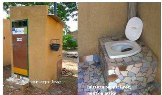
Fig. 3: Outside and inside views of a single vault UDDT constructed at town halls in Ouagadougou (with urine diversion seat) (source: CREPA, 2008).
