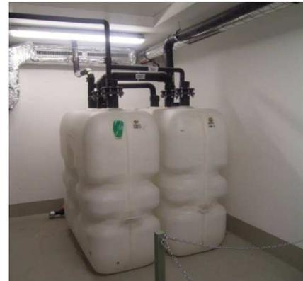
**Fig. 7:** The two plastic urine tanks (currently bypassed) in the school building's basement have a capacity of 1.5 m<sup>3</sup> each (source: OtterWasser GmbH).
