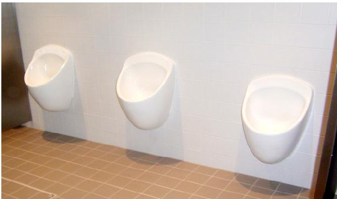
**Fig. 6:** Waterless urinals for boys from the Austrian company Hellbrok in the school building – hung lower than for adults (source: OtterWasser GmbH).
