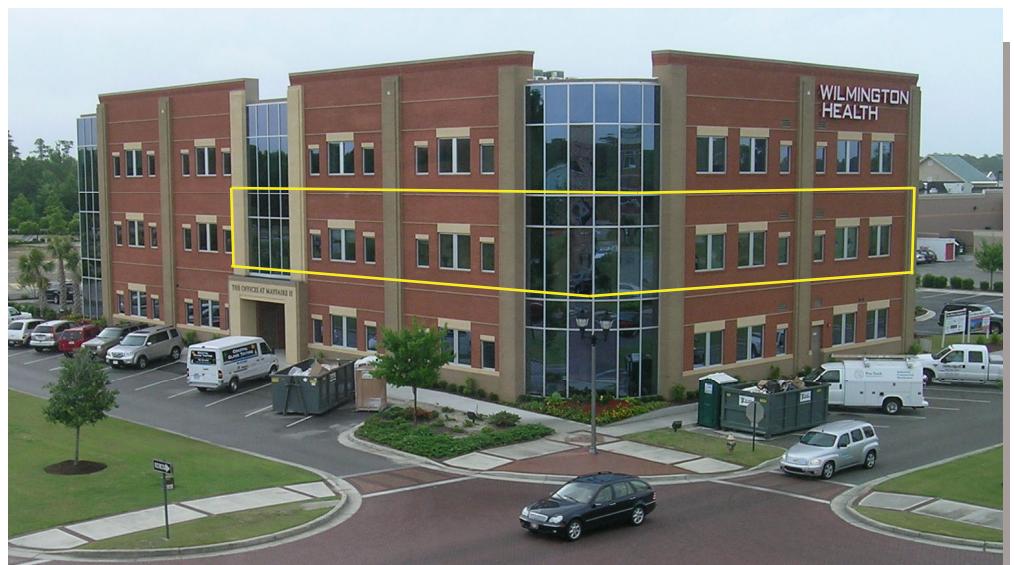
Western and Southern view of the Subject Property. The property is located on the Second Floor.
