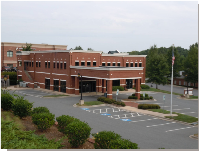
Front of Building and Covered Drop Off
