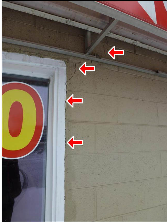
2.2 Item 4(Picture) Exterior wall shift around windows
