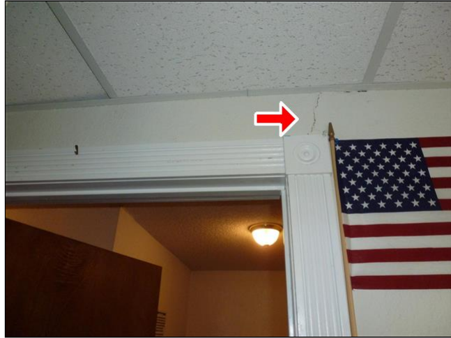
7.4 Item 2(Picture) Header crack
