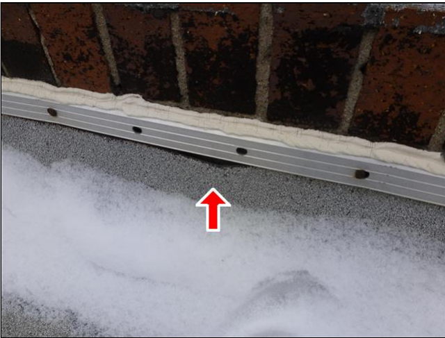
1.0 Item 5(Picture) Roof membrane loose
