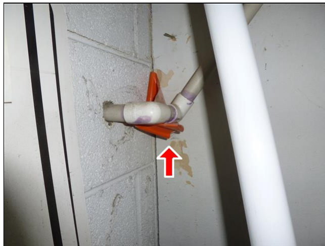
4.0 Item 4(Picture) furnace condensation drain
