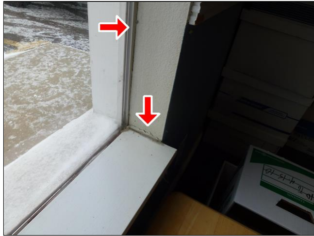
7.1 Item 2(Picture) Silicone cracked
