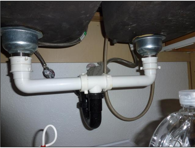
5.0 Item 1(Picture) Kitchen area plumbing drain system
