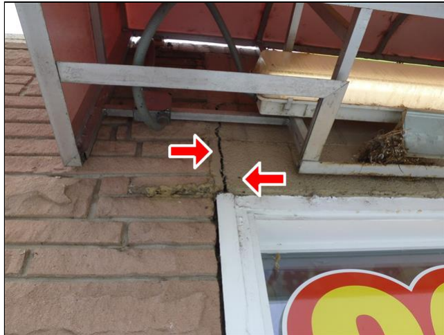
2.0 Item 6(Picture) Exterior crack above window
