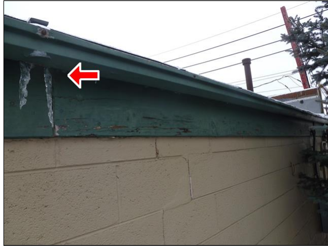
1.3 Item 2(Picture) Roof leak behind drainage system
