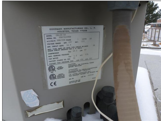
4.6 Item 2(Picture) A/C manufacture tag
