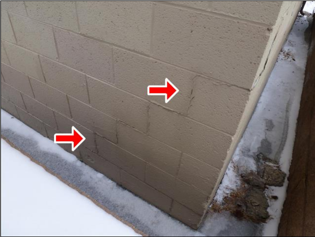
2.0 Item 3(Picture) Exterior wall shift
