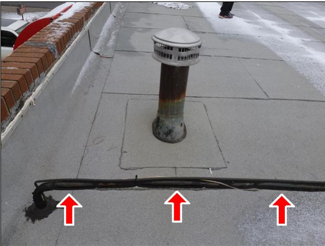
4.6 Item 1(Picture) Insulation missing
