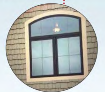
RAISED STUCCO WINDOW TRIMMING
