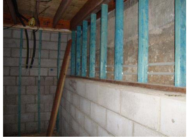
New framing in basement resulting from the expanded ceiling height.
