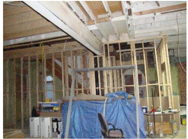
Looking toward former hotel building from bar area. All new framing.
