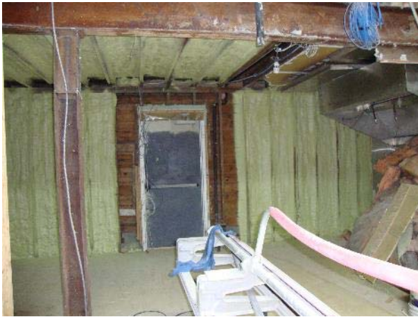
New framing and spray foam in bar area.
