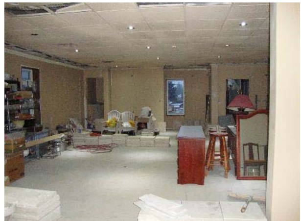
Proposed dining club on the second floor. Suspended ceiling with drywall walls. Travertine marble tiles stacked on subfloor.
