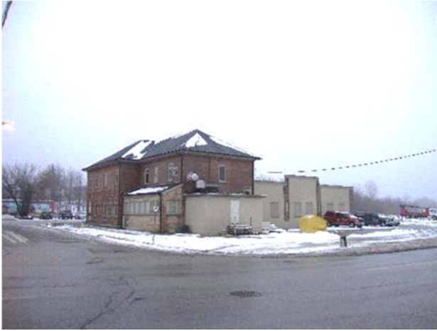
Looking northeast from Henry St & Victoria St intersection. Original hotel portion is on left site and restaurant/addition portion is on right.
