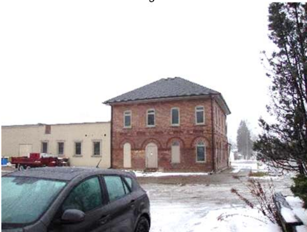
Looking south at rear of building. West property line is right edge of the sidewalk visible beside building.
