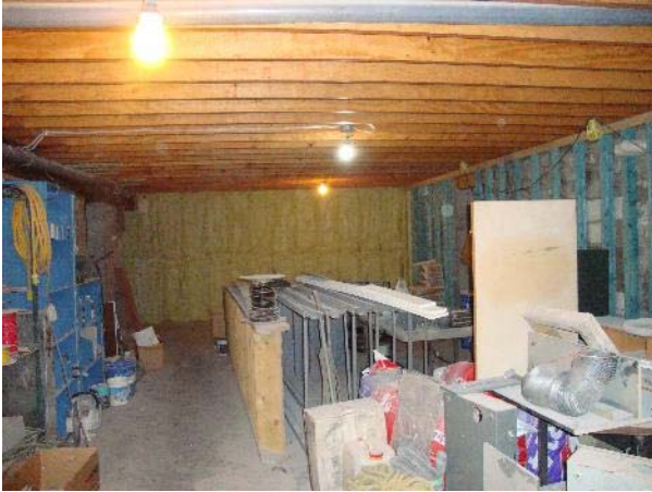
Reconstructed basement. The concrete floor was poured after the basement had been sub-excavated 2 feet.
