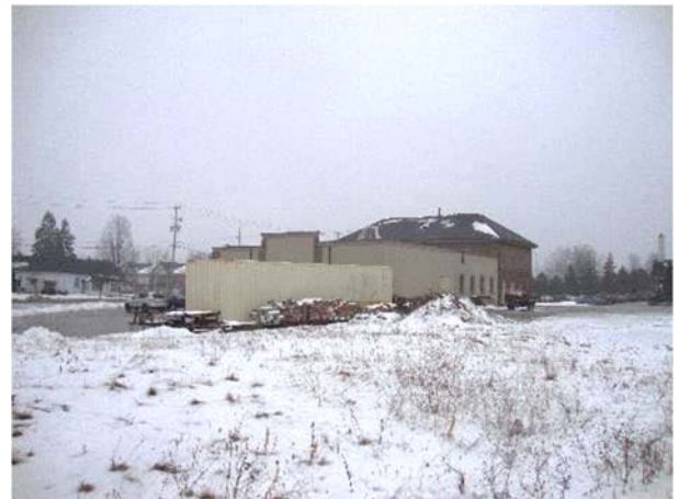
Looking southwest across small fill piles and storage 'sea can' toward building.
