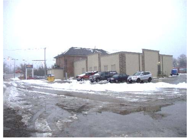
Looking northwest toward building and asphalt parking area.
