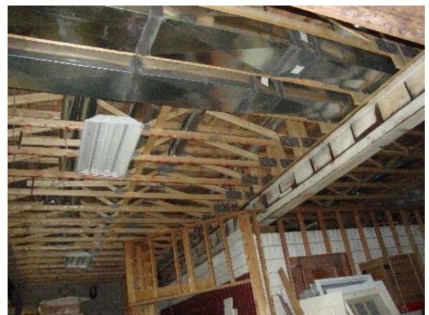
New trusses for concrete roof over bar and banquet hall area. New ducts visible.
