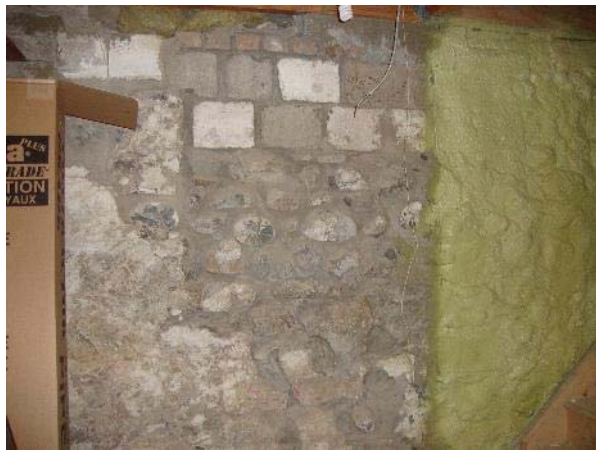
Original stone and brick foundation under the former hotel building. Note the new spray foam to the right.
