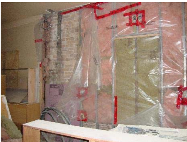
Exposed brick exterior wall on the second floor with partially completed metal stud framing.
