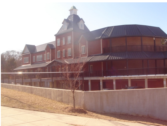
Figure 2.7 The concrete flood wall around the Takoma Park Community Center.
