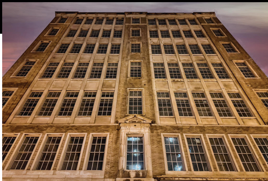
THE BELL BUILDING (FORMERLY BELL TELEPHONE EXCHANGE ) Trenton, NJ Built: 1913 Windows: Single Hung
