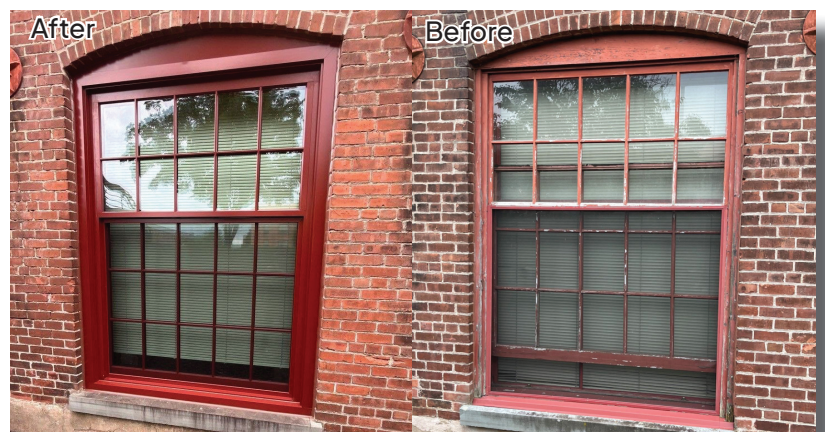
BIGELOW COMMONS (FORMERLY BIGELOW–HARTFORD CARPET MILL ) ENFIELD, CT
