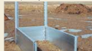
To begin assembling shield, two corner end-posts are pinned to side panels and rear panel.
