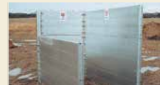
Side and rear panels are stacked to desired height.
