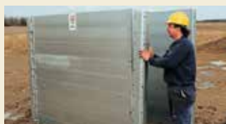
Corner end-posts are pinned in place.
