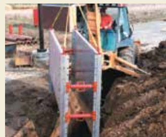
To begin assembling shield, two corner end-posts are pinned to side panels and rear panel.
