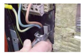
5. Install the power cord: attach the wires to the terminal block as follows:
