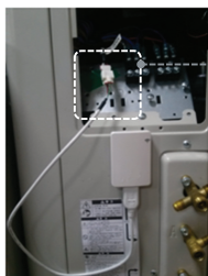
Connect module connector to outdoor unit main board FAC MVC Jig
