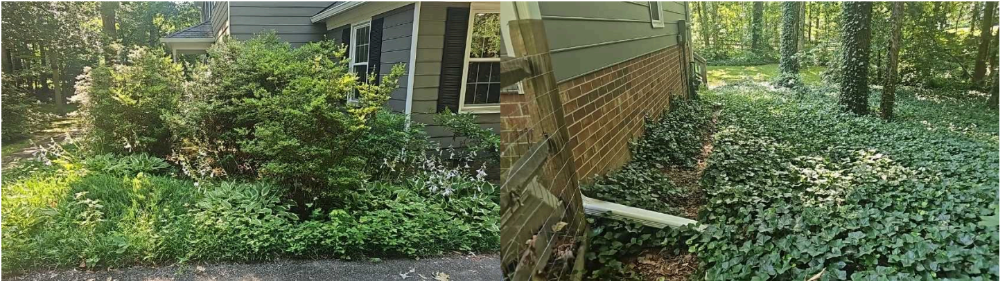
Ivy vegetation is overgrown
