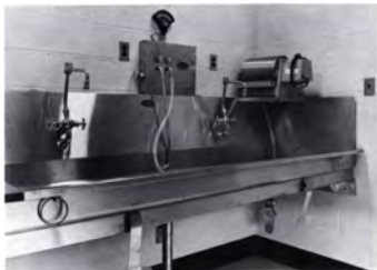
One of 16 color printing darkrooms. Wet side is equipped with Kodak CP-5 drum processor, Oscar Fisher temperature control and custom sink, and knee switches for white lights.
