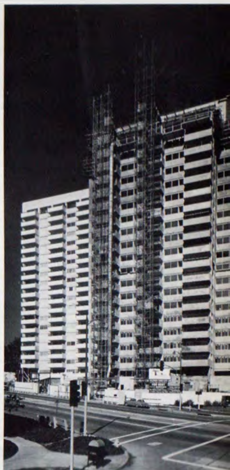
Construction nears completion as lights begin to appear in windows of first four floors.
