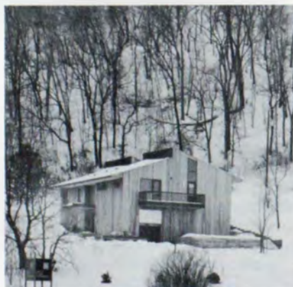
Summer and winter views of the studio's exterior. Siding is of rough sawn cedar; lights built in overhanging roof illuminate building at night. Revoir has black-topped a parking lot with space for five cars, and set up a lighted sign by the highway.
