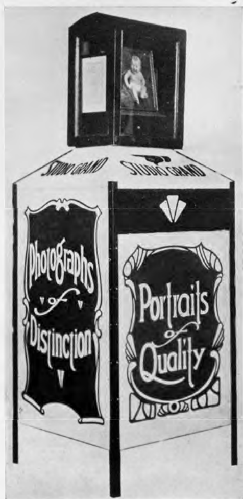
The Studio Grand, Kokomo, Ind., ran into difficulties when they wanted to install a permanent showcase abutting on the sidewalk, and the local authorities refused permission. This shows how they managed to get around the prohibition, by making a movable stand of angle-iron and beaver board, with a glass-enclosed cabinet at the top for the display and showcards.
