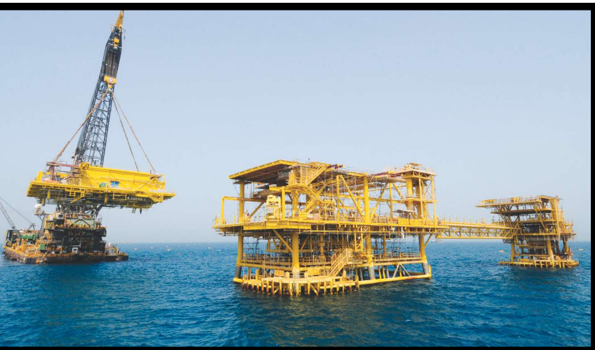
The TP-18 platform is located in the Marjan Field offshore Saudi Arabia. The EPCI contract was awarded to McDermott by Aramco earlier this year for the upgrade of two existing platforms. (Source: McDermott)
