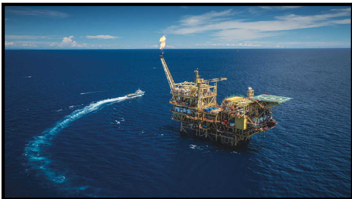
PETRONAS' Semarang offshore platform s located off the coast of Terengganu, Malaysia. (Source: PETRONAS)
