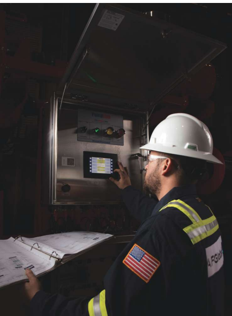
The AMI Controls & Analytics group offers complete end-to-end hydraulic pressure pumping control automation and data management through its FracCommand Suite. (Source: AFGlobal)
