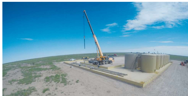
The MPS is an integrated field facility installed between the well and the pipeline for oil and gas processing applications. (Source: Tri-Point Oil & Gas Production Systems)
