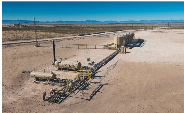
A MPS accommodates single-well to multiwell layouts, offering plug-and-play capabilities and life-of-well flexibility.
