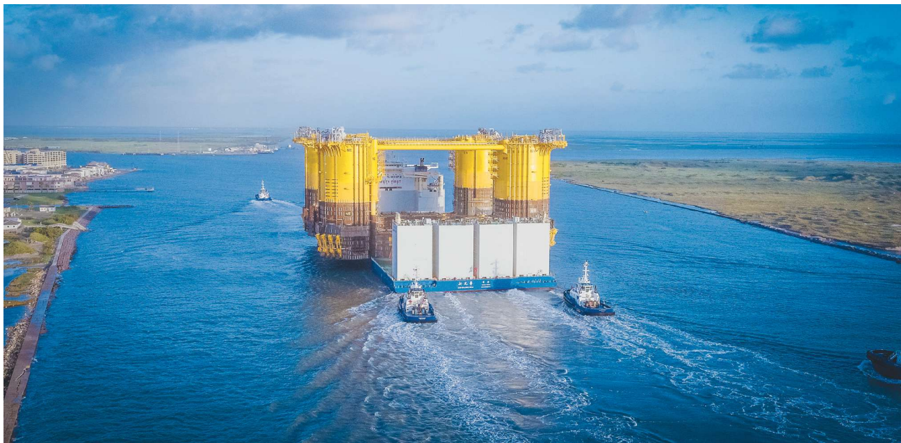
For the Appomattox Field development program, Shell was able to take 25% of cost out after the FID. (Source: Shell)
