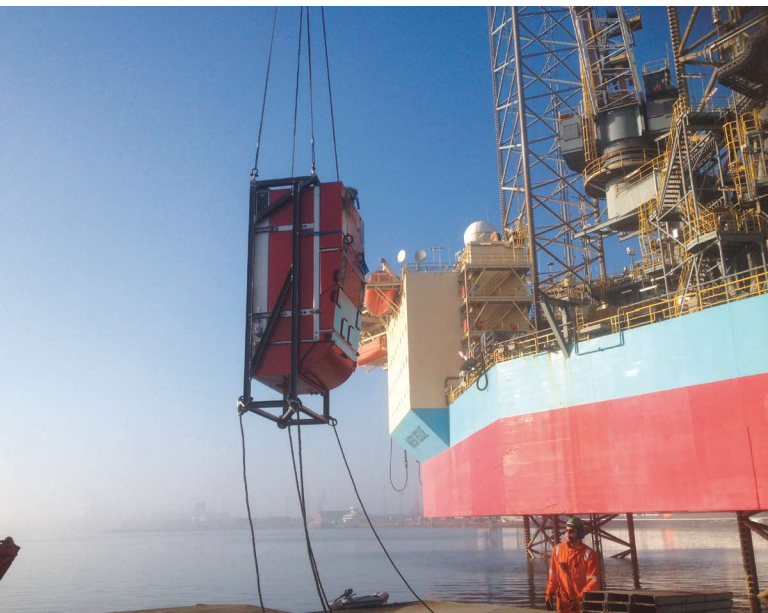
Cubility's MudCube is installed on an offshore rig. The system provides lower fluid consumption and reduced waste volumes. (Source: Cubility)
