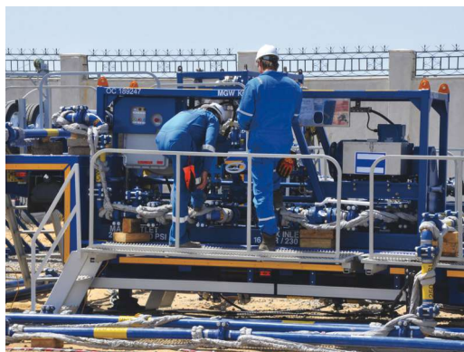
Maintenance technicians perform routine inspections at a job site. (Source: photostock77, Shutterstock.com)
