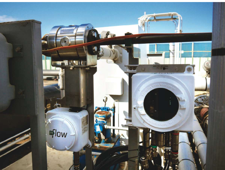
The carbon fiber construction of an M-Flow metering system makes it possible to deploy sensor systems fully protected from aggressive oil well fluids. (Source: M-Flow)
