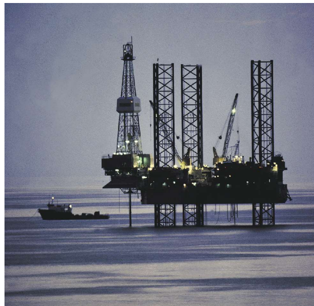
Corrosion, condensation and freezing are major issues on a cold-stacked rig. (Source: Aggreko)
