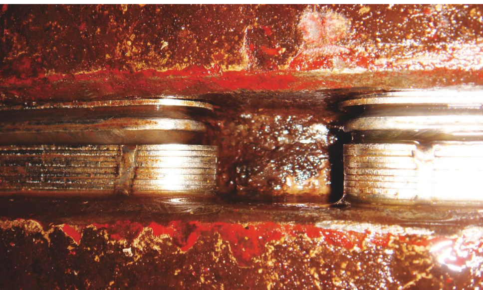
ThinJacks sandwiched within matching ThinShims are placed exactly where the force is needed, exerting 328 tonnes of force. (Source: ThinJack Ltd.)
