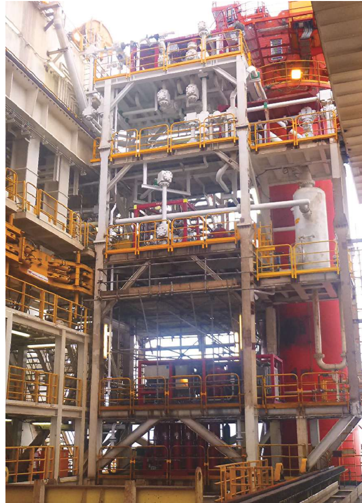
MPD equipment (in red) is installed throughout the decks of the drillship. (Source: Halliburton)
