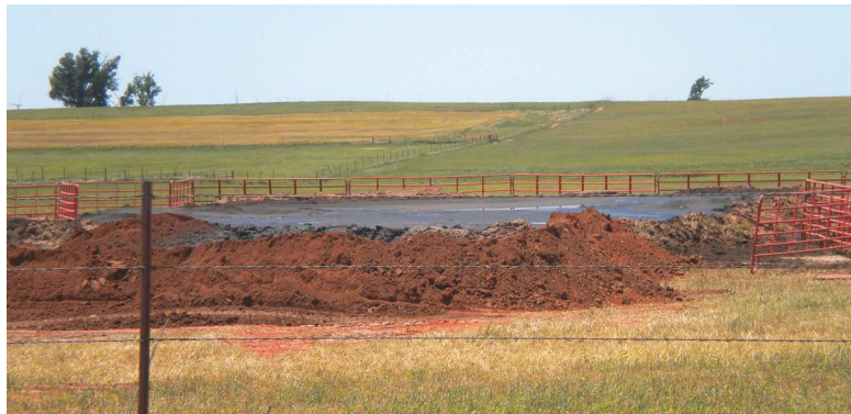
Drilling waste containing diesel-range organics and other constituents is being stored at a receiving site prior to landfarming. (Source: Scott Environmental Services)
