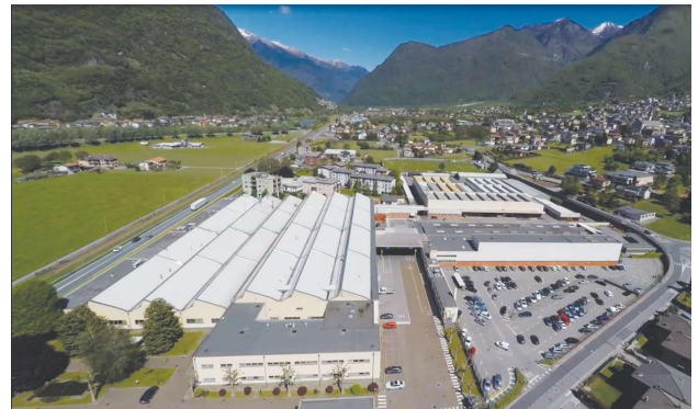
The GE Oil & Gas facility in Talamona, Italy, has two high-tech component production lines. (Source: GE Oil & Gas)
