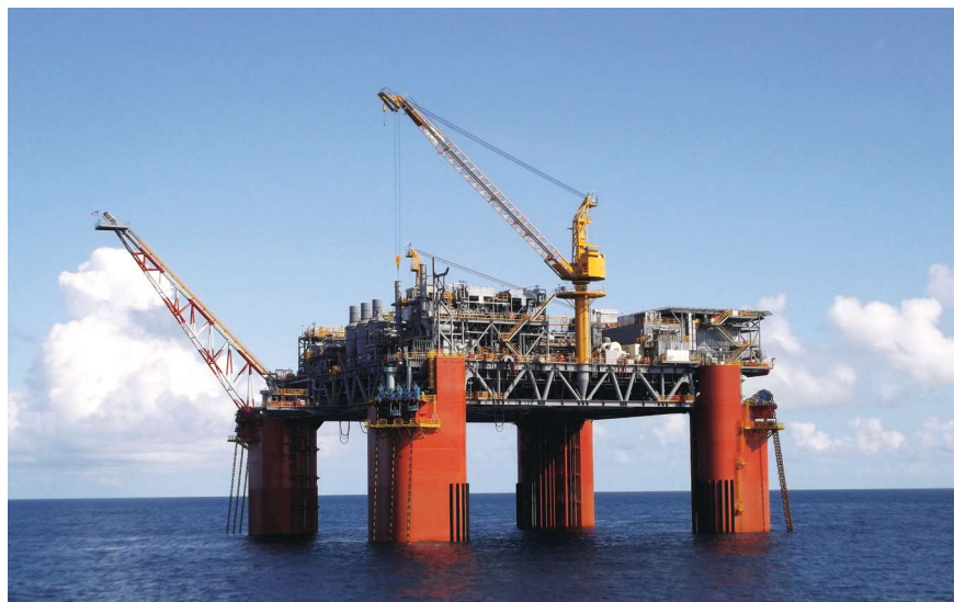
Engineering work for the Delta House facility began before the discovery well was drilled. (Source: LLOG)
