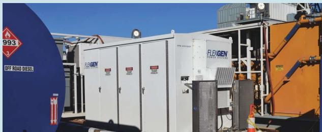
The FlexGen Solid State Generator reduces capital costs by decreasing the size and number of generator sets and alternators required to support load demand. (Source: FlexGen Power Systems)
