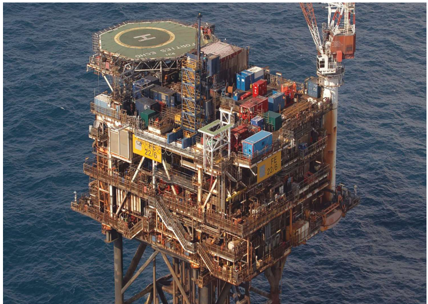
The Forties Echo platform originally had a small workover rig on skid beams. The drilling derrick, drill floor and beams were removed from the platform. The Galaxy III rig was jacked up next to the platform in early 2004 to start sidetracking wells. (Images courtesy of Apache Corp.)
