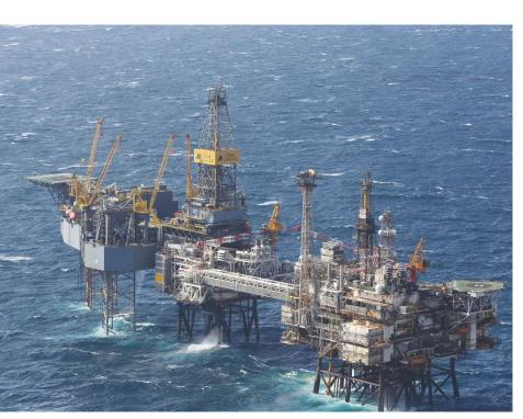
The bridge-linked FASP (left) was installed in 2014 by operator Apache to work in tandem with the original Forties Alpha Platform. (Source: Apache Corp.)
