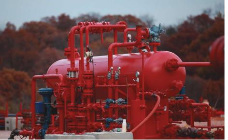
Test separators efficiently remove oil and gas from flowback and produced water. (Source: Select Energy Services)
