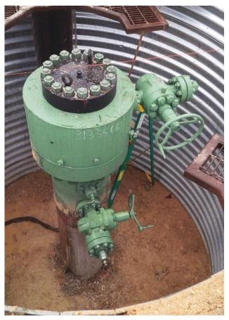
The nested design of the MN-DS wellhead allows the whole system to easily fit under most skidded drilling rigs. The system can be installed along with all subsequent strings through the diverter riser/BOP. (Source: Cameron)
