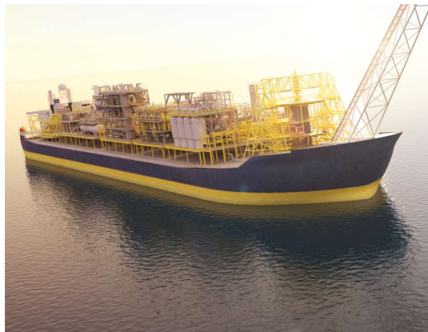
A typical FPSO topsides structure shows the finite amount of expensive real estate available. (Source: Cameron)
