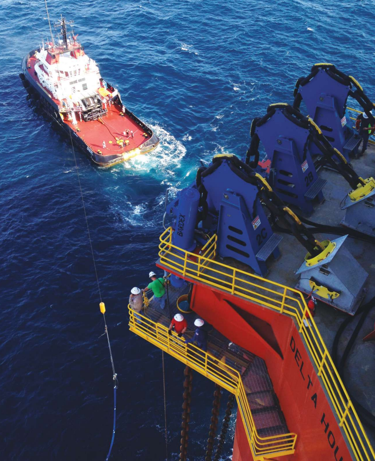
Chain-reaction: LLOG Exploration's Delta House semisubmersible production platform was installed on the field in Mississippi Canyon Block 254 in October 2014. It is permanently moored via 12 preset chain/polyester mooring lines. The system, which also includes 12 suction pile anchors, was designed, fabricated, installed and hooked up in 1,356 m (4,450 ft) of water by Acteon subsidiary InterMoor. (Source: InterMoor)
