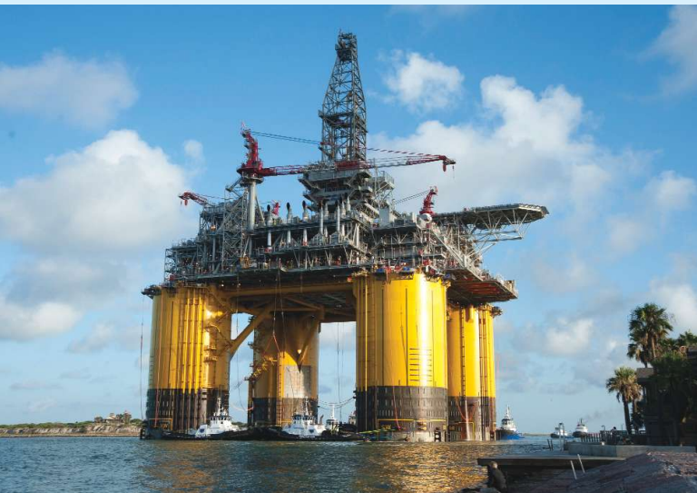
The tow-out and transportation of the platform used for the first time ever synthetic rigging rather than traditional steel wire rope. (Source: Shell)
