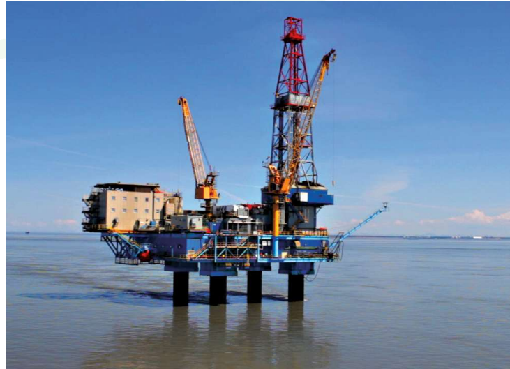
Miller Energy Resources' Osprey platform is 5.6 km (3.5 miles) southeast of the Kustatan production facility in Cook Inlet. The platform sits in 18 m (60 ft) of water and is designed for 21 wells producing 25 Mbbl/d of oil. (Source: Miller Energy Resources)
