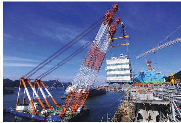
The first topsides module weighing 2,000 tons is lifted into place on the *PFLNG1* FLNG facility at Daewoo Shipbuilding & Marine Engineering's yard in Okpo, South Korea. A further 20 modules weighing approximately 40,000 tons remain to be installed, with the facility (to be named *PFLNG Satu*) due for completion by year-end 2015. (Source: Petronas)
