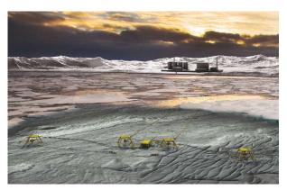
A conceptual rendering shows a subsea production system in an arctic setting similar to the one deployed in the Kirinskoye field off the coast of Sakhalin Island. (Image courtesy of FMC Technologies)
