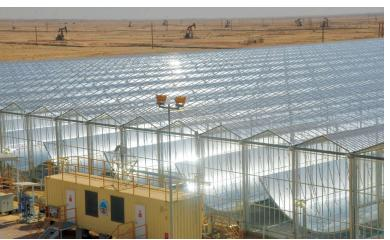
This solar EOR operation in the Amal West oil field in southern Oman takes up four acres. The glass houses protect the sensitive mirrors and solar technology from the harsh elements. (Images courtesy of GlassPoint Solar)
