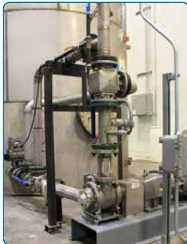
The clean room at the new EMCO facility utilizes a stainless-steel SNP Series Sliding Vane Pump to transfer chemicals with unique handling characteristics.
