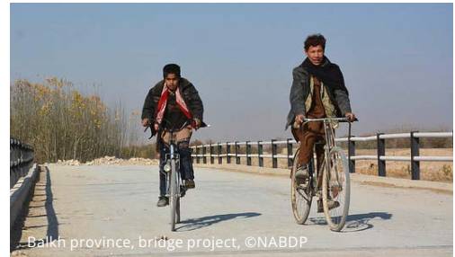
Balkh province, bridge project, ©NABDP
