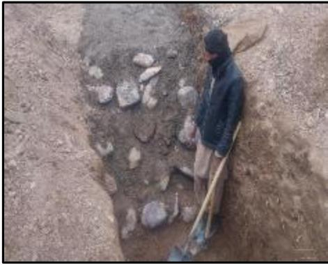
During a monitoring visit of PMT team to Nahr-e-khejak village of Adraskan district in Herat province to monitor the progress of (2.45 Km) Protection wall. The monitoring team discover some problems in the usage of construction materials in the foundation of protection wall; the construction company used the river stone instead of using construction stones in the foundation of wall. Which was reported to the project manager, and taken in consideration and solved accordingly.
