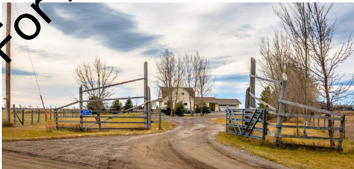
Gated north property entrance approach and the existing dwelling beyond. Lethbridge, Alberta
