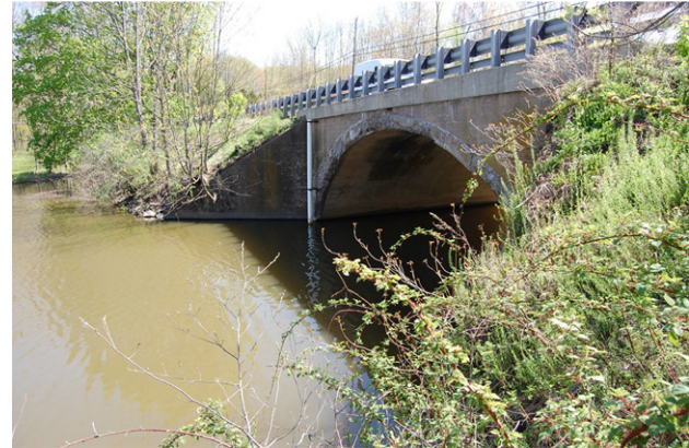
Threemile Run flows through arch culvert beneath PA Route 313
