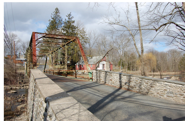
Nursery Road historic through-truss bridge over Unami Creek
