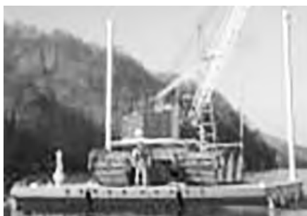
32' x 40' x 4' Sectional Spud Barge and Crane.
