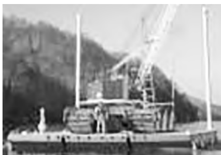
32' x 40' x 4' Sectional Spud Barge and Crane.
